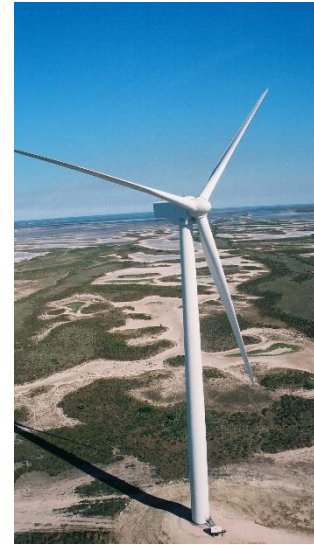
Clean / Renewable Energy
